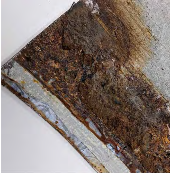
Figure 1: Zintec mild steel showing galvanic corrosion
